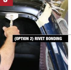
Clamp panel in place. Do not over clamp. Install rivets or STRSW per manufacturer's recommendations during adhesive's working time. Remove clamps after rivets or spot welds have been installed on panels fully supported by these methods. Wipe away excess material.
